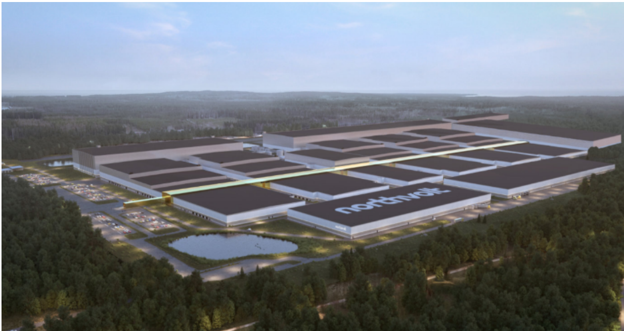
An artistic impression of Northvolt's first factory to be established in northern Sweden. (Credit: Northvolt)
